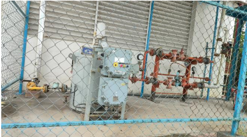
LPG Vaporizer re-located
